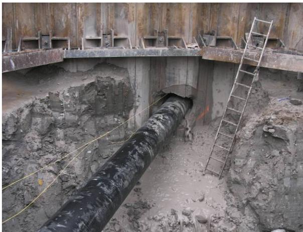
Figure 6 HDPE Pullback
