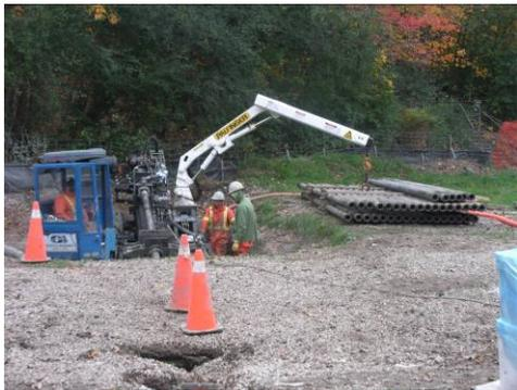
Figure 2. Machine Cut below grade to accommodate short distance to MH
