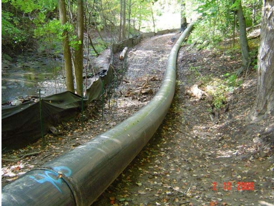
Figure 1 – 635m of 600mm HDPE Sunnybrook Subtrunk on Grade Installation 2006
