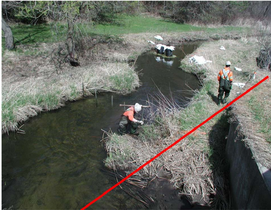
Figure 4 – Bore path(red line) and frac control measures
